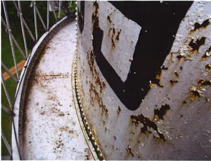
Tank shell coating typical
