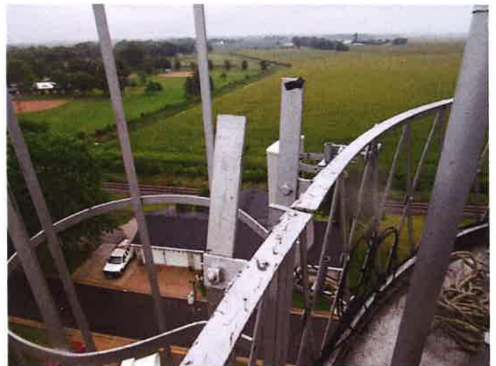
Ladder needs walk thru as per OSHA
