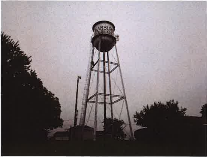
Exterior over view of water tower.
