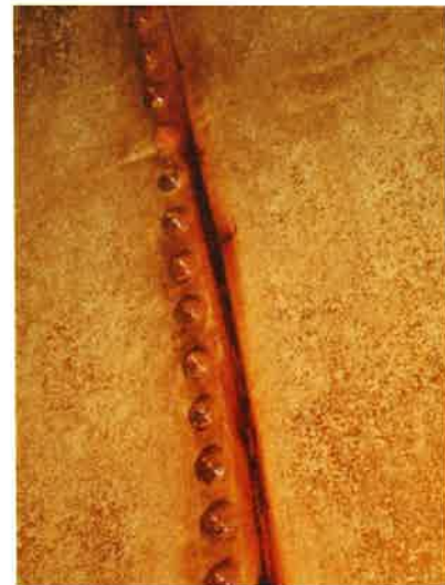
Corroded lap seams in the belly
