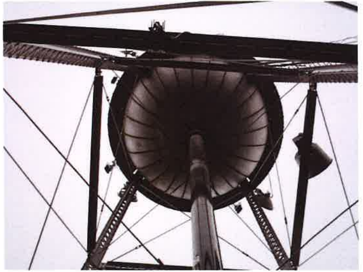
Looking up at belly of water tower
