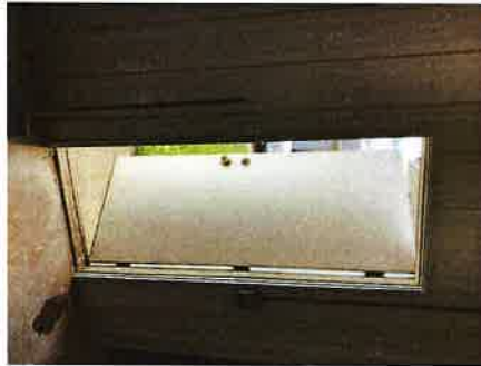
WELL HOUSE/FILTER ENTRANCE DOOR
